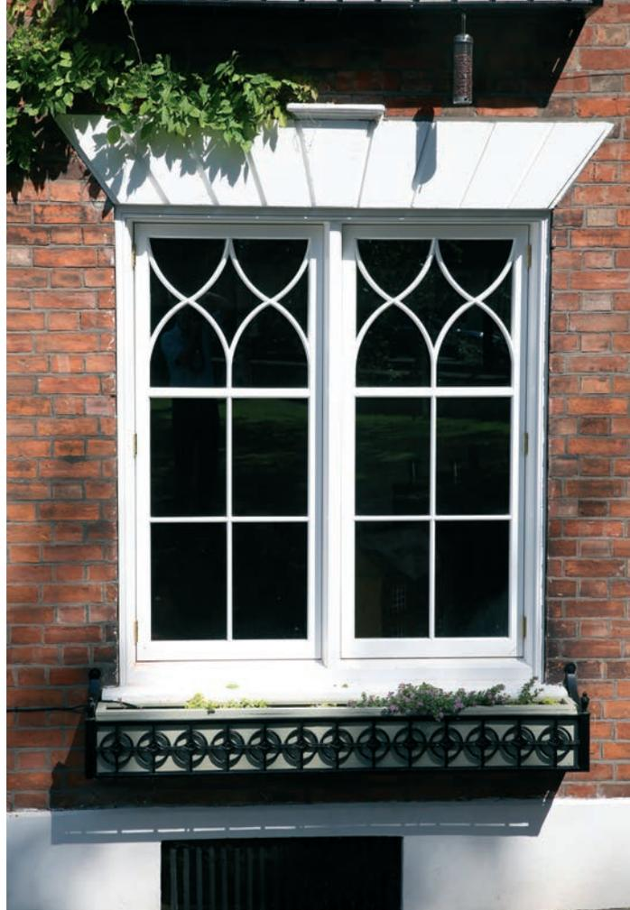
achieved by creating a hole in the inner pane, which is located 50 mm from the edge of the glass and covered by a permanent 12 mm black plastic cap. For some conservation officers this can be a distraction, but for many others it is barely noticeable behind the curtain sweep. Similarly, the 0.25 mm micro-spacers, which sit at 20mm intervals to keep the two panes a fixed distance apart, are visible on close inspection, but not in day to day use.
